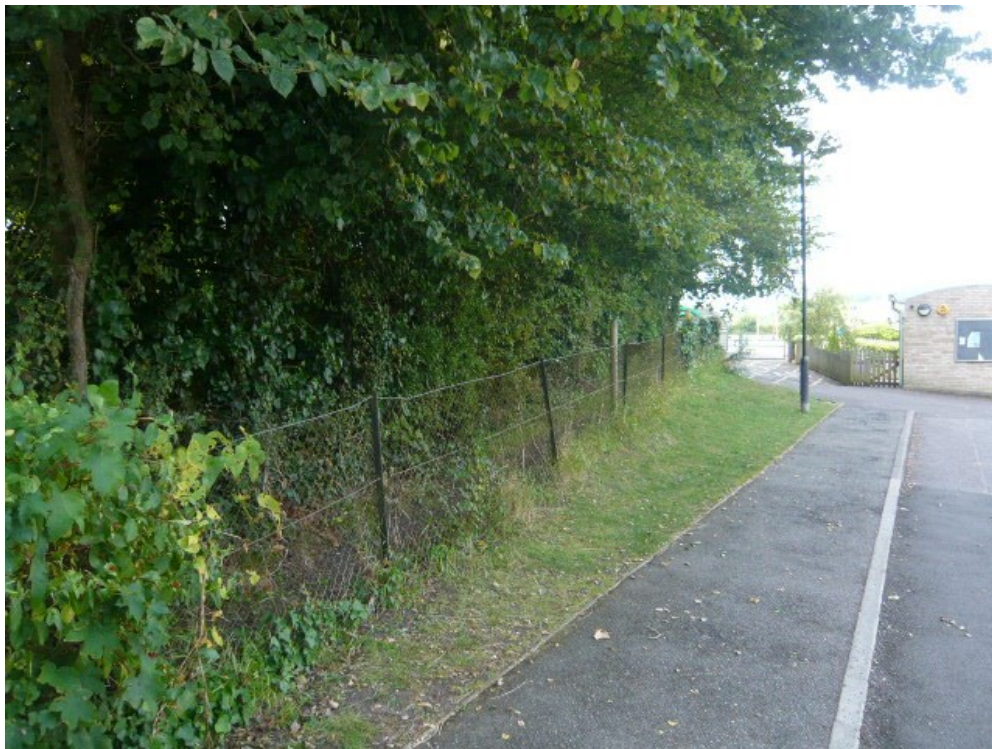
9: Existing low chain link fencing to be replaced with 1800mm high weld mesh fencing to improve safeguarding adjacent to diverted public Right of Way FP62.
