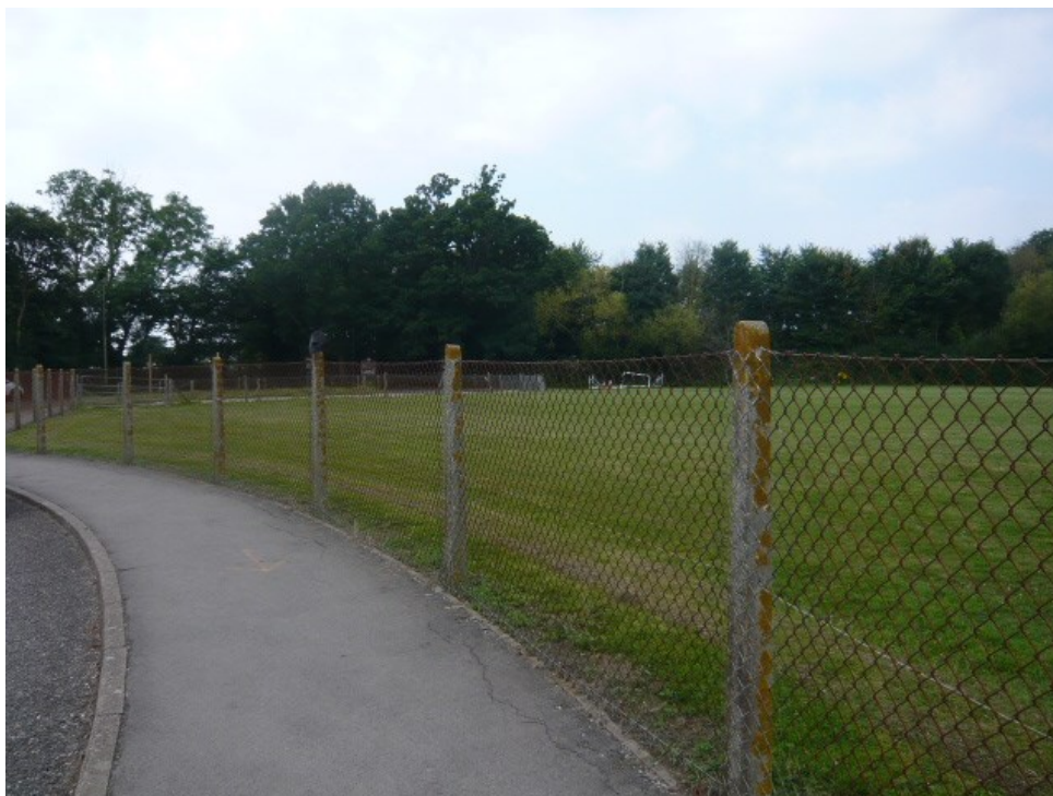
7: Existing fence to Playing Field perimeter to be replaced with 2100mm high weldmesh fencing. Gates to be installed for grounds maintenance.
